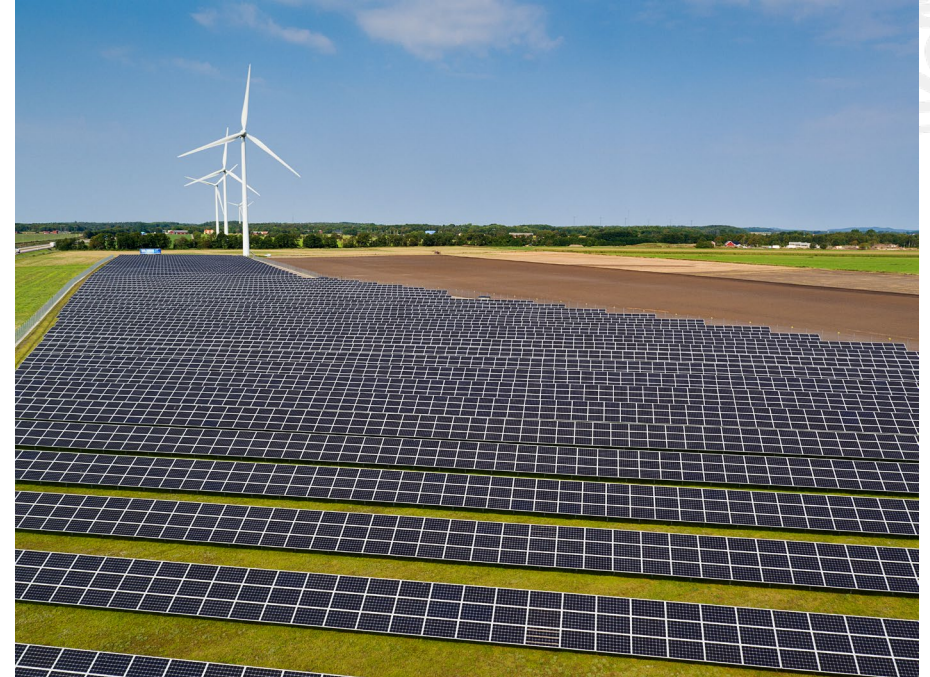
Example of co-located wind and PV park in Sweden [Source: Thomas Carlén].
